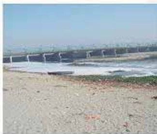
Downstream of Okhla Barrage - located 2.5 kms d/s of old Okhla Weir with a design flood of 3 L cusecs. Pond level is 201.35 m with upstream bed level at 194.85 m and d/s bed level at 194.45m. Water is diverted to Agra Canal (4000 cusec) and Gurgaon Canal (2240 cusec) just before the barrage
